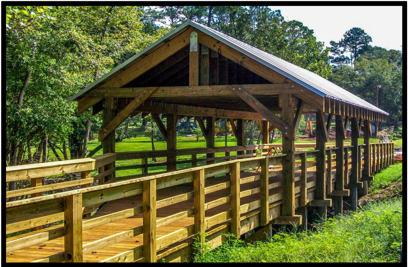
Silverhill Sidewalk Improvements – Silverhill, Alabama: 50' LF of 8' Cart Bridge, 75 LF of 8' Cart Bridge, 40' LF of 8' Cart Bridge and 110 LF of 12' Cart Bridge
